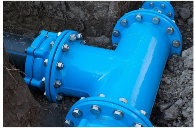
Figure 16. Bolt-on flanged pipeline system
