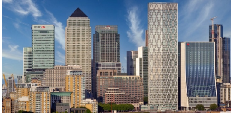
Şekil 4. Canary Wharf ( https://group.canarywharf.com/about-us/ , t.y.)
