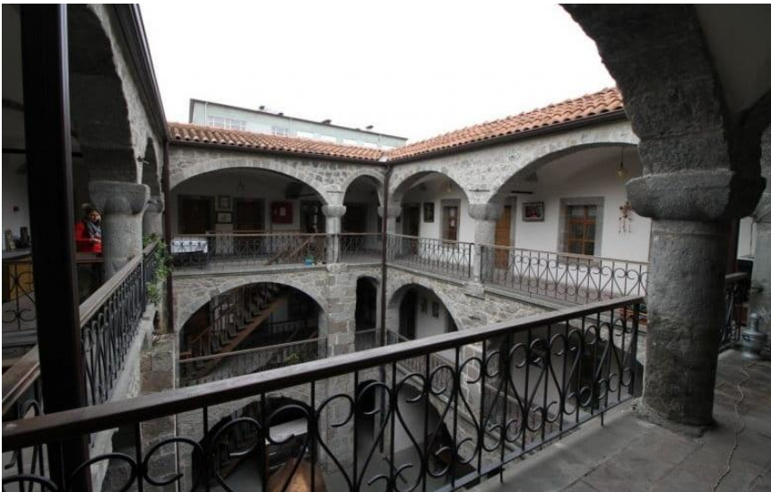
Figure 2: Interior of Alaca Han after restoration (Source: Karadeniz Kültür Envanteri)
