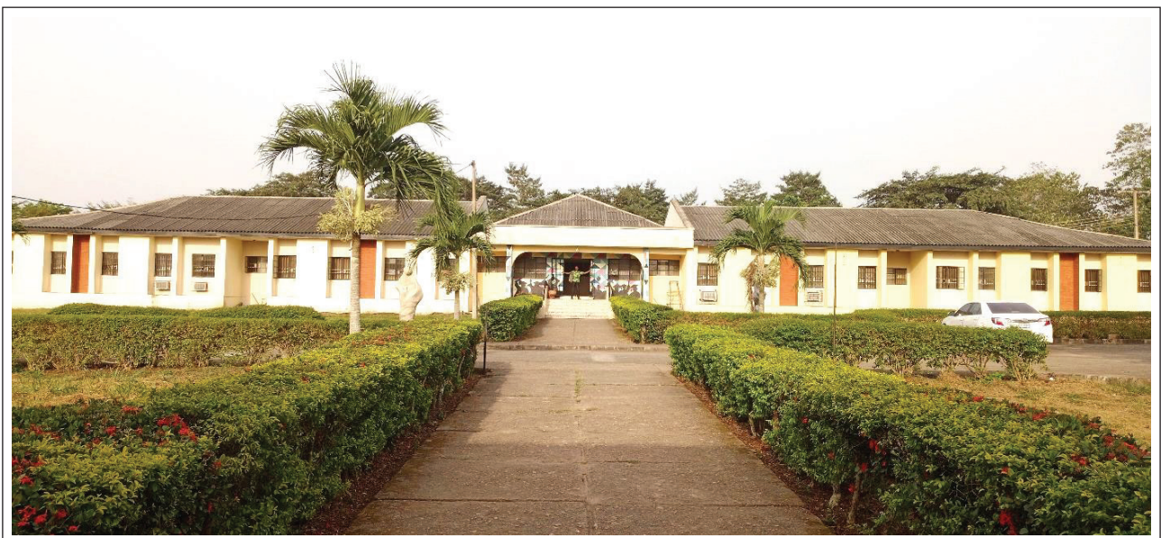
Figure 2. A fullview of the Fine and Applied Art Department Building (© Siyanbola Afeez 17/12/2021).
