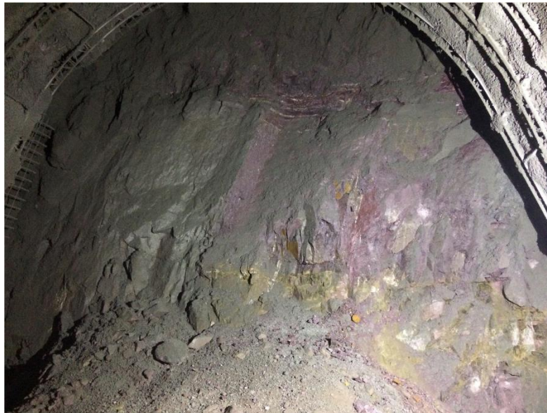
Figure 2. Tunnel face in Kurtköy Formation in M5 metro line Umraniye station
