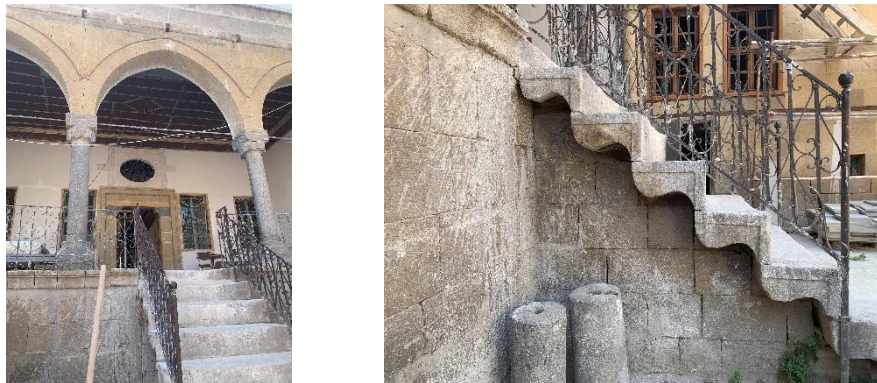
Figure 9. Profile detail of the stone steps leading to Hanay (author archive, 2022)
