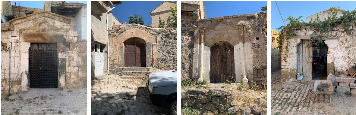
Figure 12. Garden entrance door examples (author archive, 2022)
