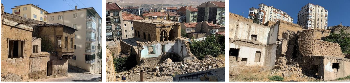
Figure 22. Kayabasi District under the pressure of apartment building (author archive, 2022)
