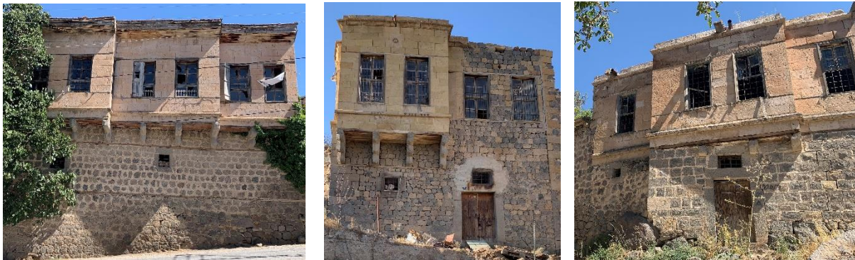
Figure 3. Traditional Nigde houses in Yesilburc Village, (author archive, 2022)
