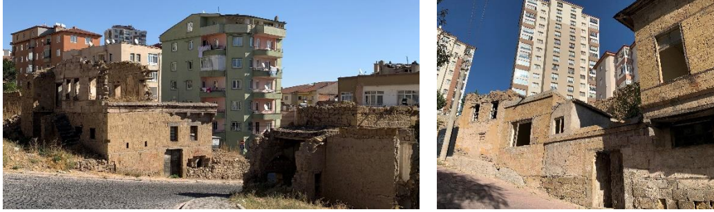
Figure 23. Kayabasi District under the pressure of apartment building (author archive, 2022)
