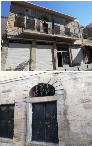
Figure 2. Epigraph of 1958 on the adjacent buildings
