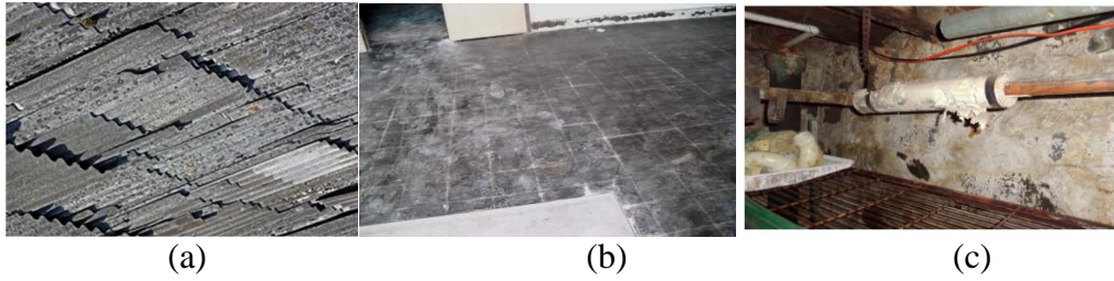
Figure 4. (a) Asbestos roofing, (b) Asbestos floor covering, (c) Asbestos pipe (Şahin ve Bingöl, 2022; Tezcan, 2007, T.C. Ministry of Labor and Social Security, 2023)
