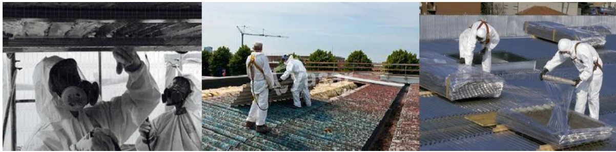
Figure 5. Examples of asbestos removal operations at the construction site (Keleş, 2022; TekMerkez OSGB 2022; EMC, 2022)
