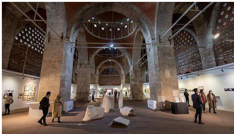
Figure 3. Tophâne- i Amire Interior, columns carrying domes (Milliyet, 2021)
