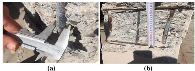
Figures 4a and 4b. Images of the reinforcement identification processes
