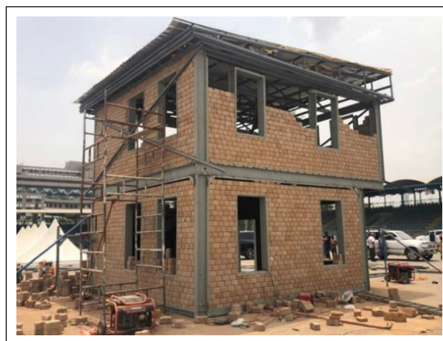
Figure 3. The ongoing building construction using ICSEB.
