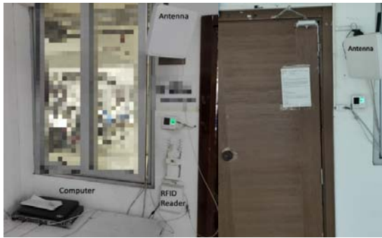
Figure 6. Testbed photographs from both sides of the gates
