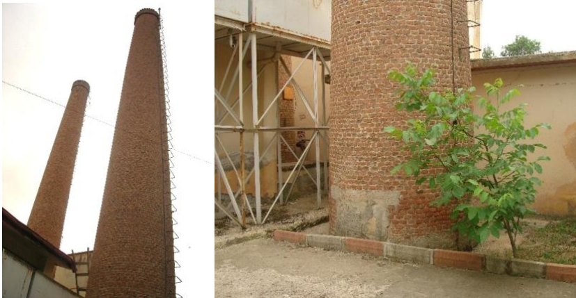
Figure 16: 1958 Gülbirlük İslamköy Rose Oil Factory Chimneys.
