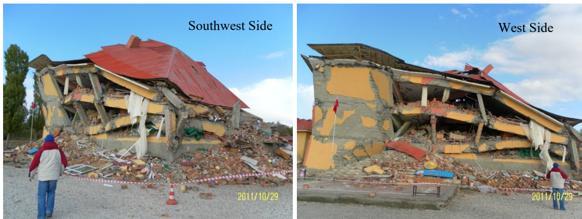
Figure 3. Southwest and west side views of the building.
