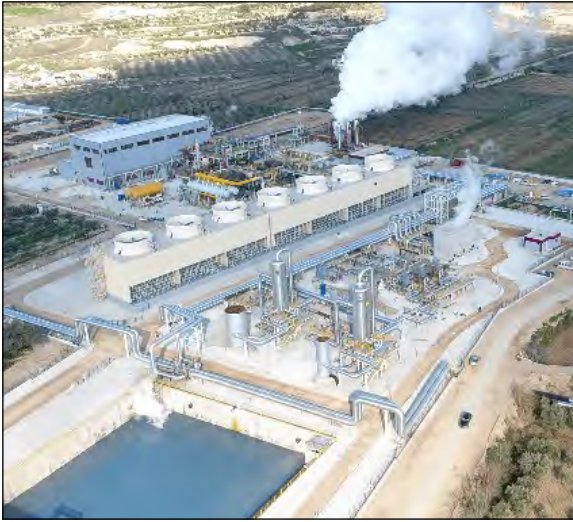
Figure 10- Kızıldere-3 Geothermal Power Plant by Zorlu Enerji Inc. in Denizli-Kızıldere geothermal field.
