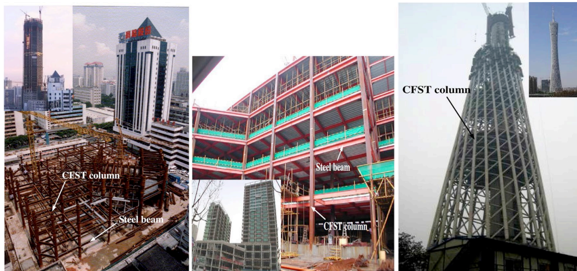
Figure 1. Some examples of buildings whose construction has been completed are in order from left to right, SEG plaza in Shenzhen, Ruifeng building in Hangzhou and Canton Tower [7]
