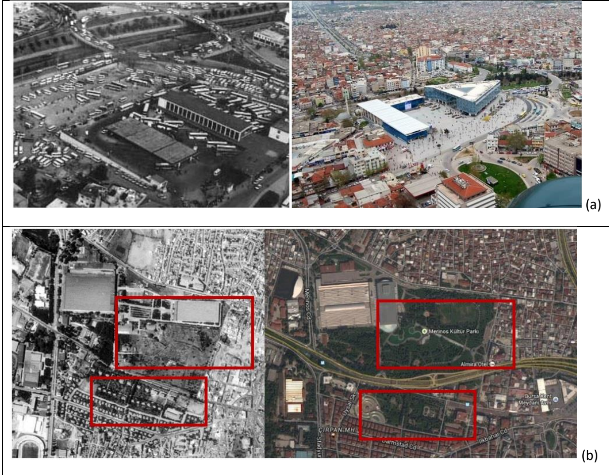
Figure 17. Before and After the Urban Regeneration Projects and Urban Design Projects in (a) Central Bus Terminal (Santral Garaj), (b) Merinos Silk Factory and its surrounding landscape
