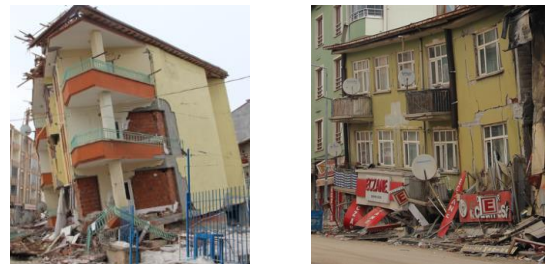
Figure 24. Collapsed structures due to sudden stiffness changes on the ground floor.
