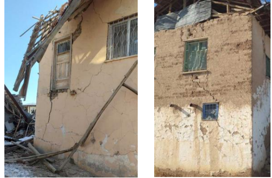
Figure 27. Shear cracks in masonry buildings
