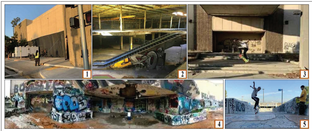
Figure 6. The current state of the building and its re-activation practices: movie set, graffiti art, and skateboarding 1-2-3-4-5 [35].
