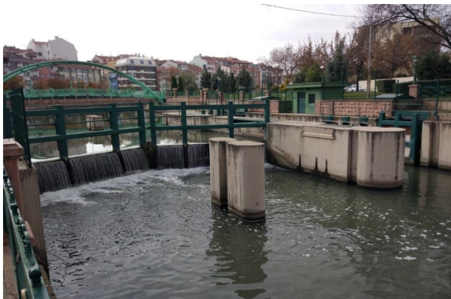
Figure 3. One of the river regulators in Porsuk Stream channel
