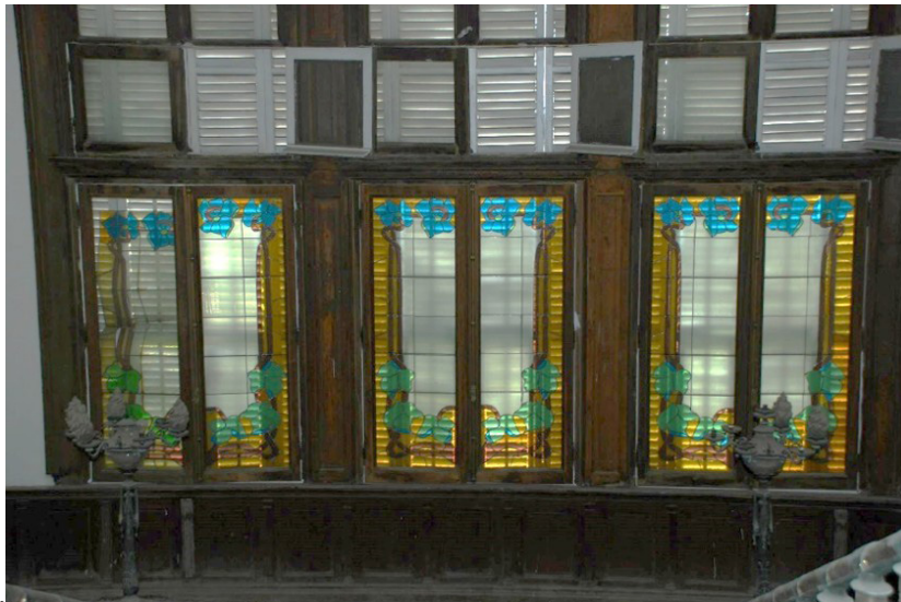
Figure 12. Ahmed Ratib Paşa Mansion window glass detail 4
