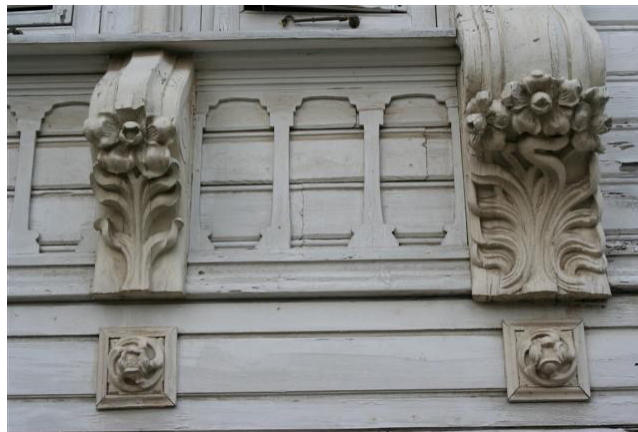
Figure 9. Ahmed Ratib Paşa Mansion Detail from façade (Aktur, H. 2008)
