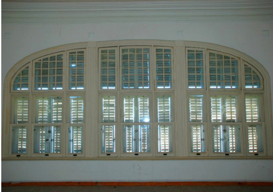
Figure 22. Ahmed Ratib Paşa Mansion roof window frame detail 10
