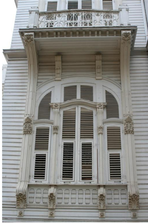
Figure 8. Ahmed Ratib Paşa Mansion Detail from façade (Aktur, H. 2008)
