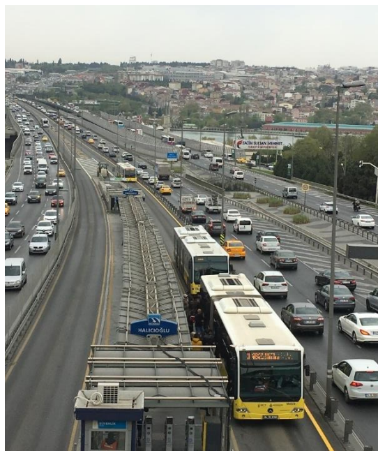
Figure 1. Istanbul BRT System
