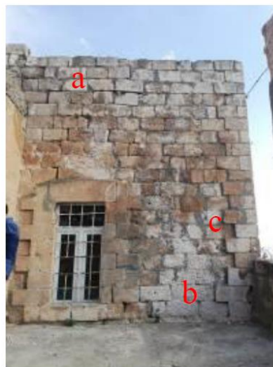
Figure 13. a. Efflorescence b. Use of cement c. Discharge of jointing d. Plant formation (Karataş,2022)
