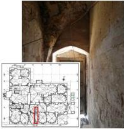
Figure 17. Colour change on the arch, tear on the sill (Karataş,2022)
