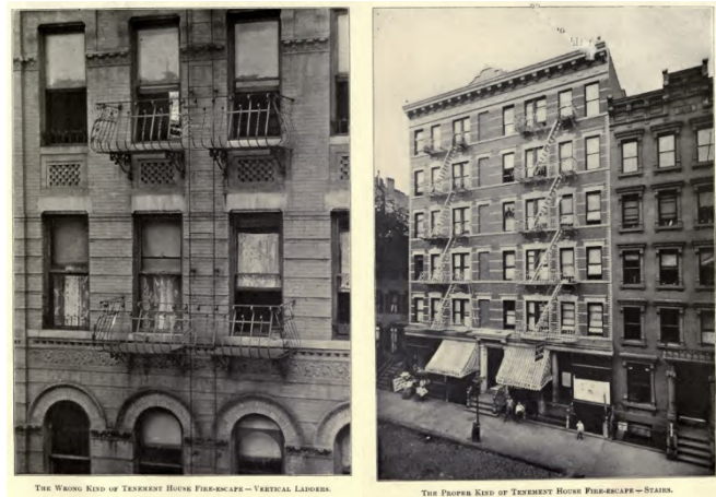
Figure 14. Fire escape balconies before the 1901 law and “Z-shaped metal stairs” after the act. (DeForest & Veiller, 1903a; p.278 & 287)
