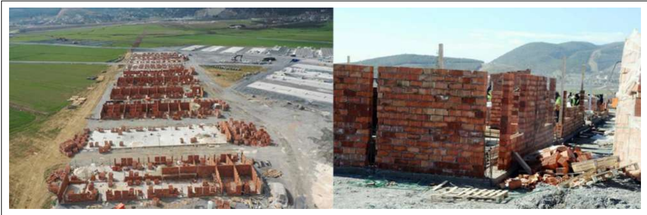
Figure 6. The construction of brick houses as temporary shelters in İslahiye [15].
