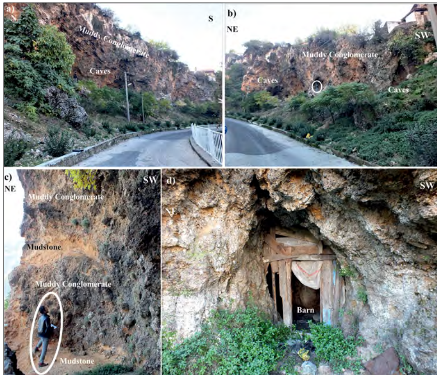
Figure 5- a) General field view of the caves on skirts of the Asar Hill, b) there are two-storey houses above the levels where the caves are located (man for scale in circle: 1.8 m), c) caves are observed in mudstone and muddy conglomerates of the Yatağan Formation (man for scale in circle: 1.8 m), d) some caves have been used as a barn for small animals.
