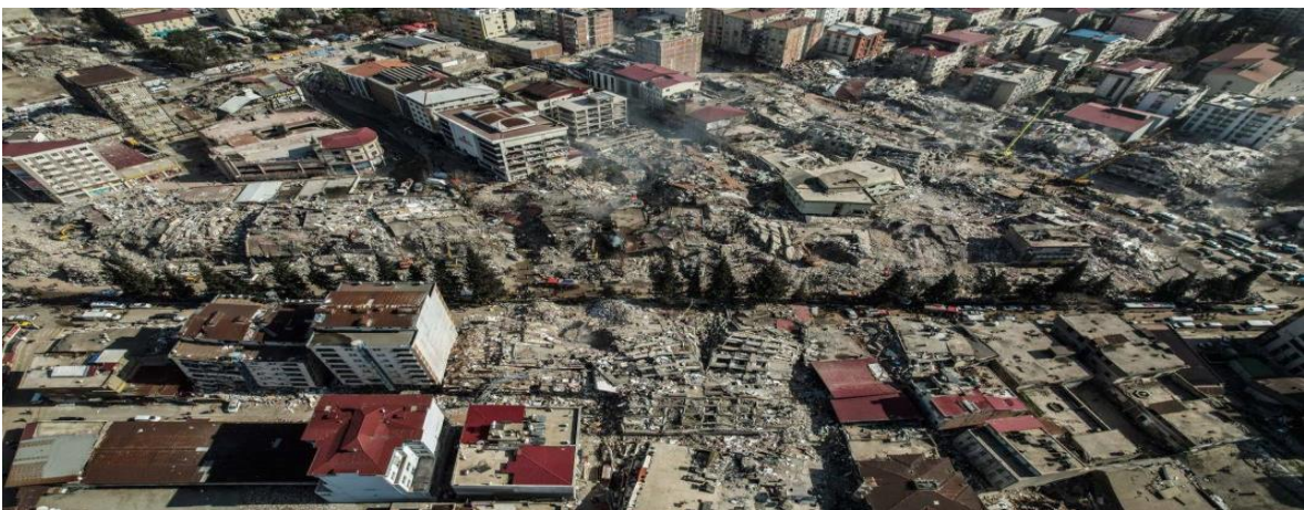
Figure 2. Images of collapsed or destroyed houses after two earthquakes in Kahramanmaras
