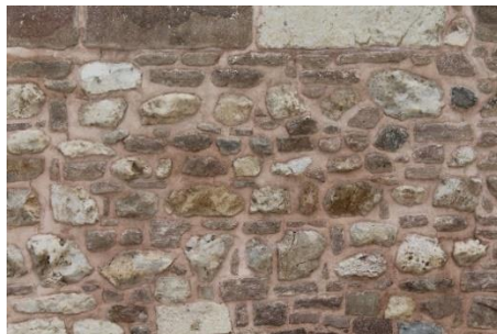
Figure 5. Grouting with hydraulic lime added horasan mortar
