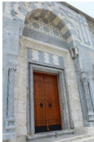
Figure 9. North courtyard gate after repair
