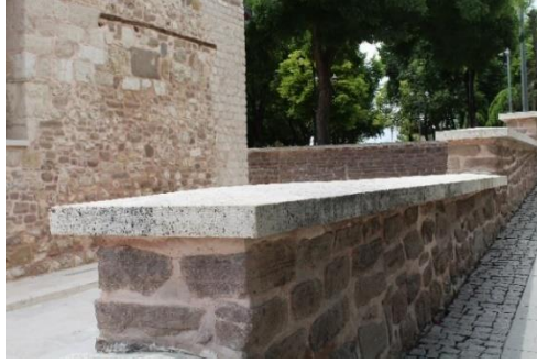
Figure 6. Addition of roofed capstone to rubble stone wall
