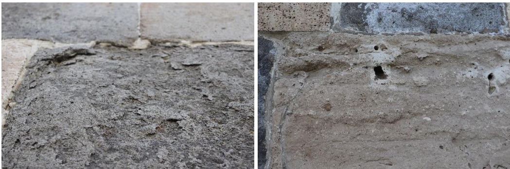
Figure 17. Abrasion on stone surface
