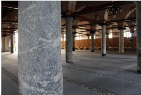
Figure 7. Surface cleaned marble columns
