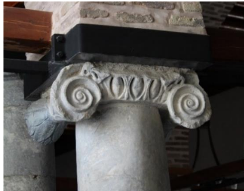
Figure 8. Column headers after repair
