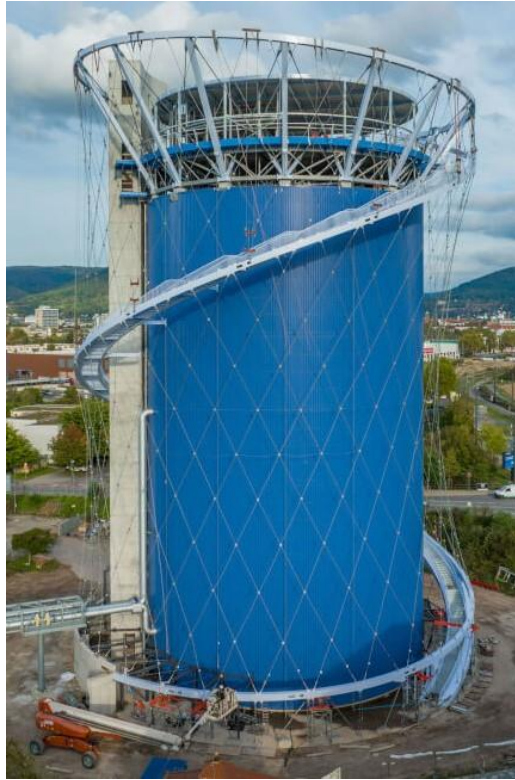
Fig. 4. Energy Storage Center (Stadtwerke Heidelberg-Model) (Germany) [25].
