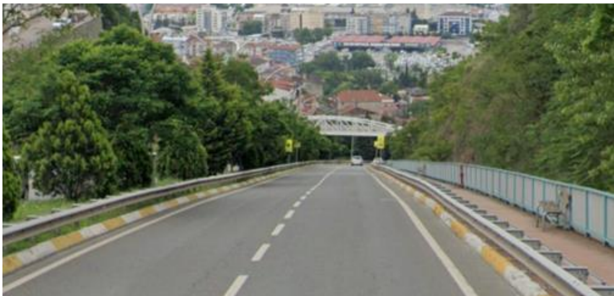
Figure 11. Work 2 sample google street view image.
