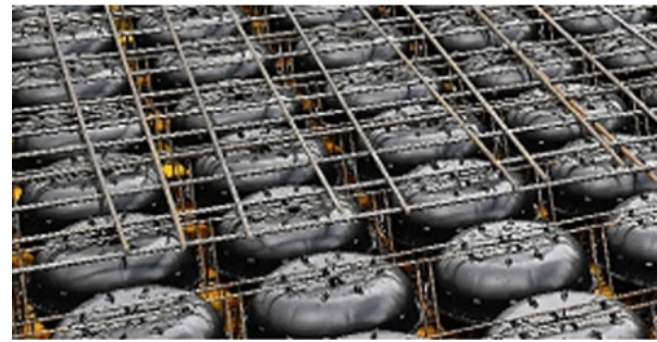
d) Cobiax slab modules and their positions
