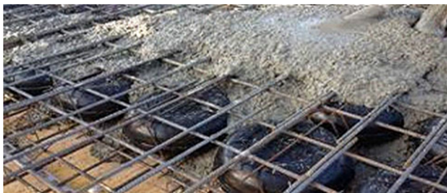
Figure 7. Concreting on Cobiax modules [11].
