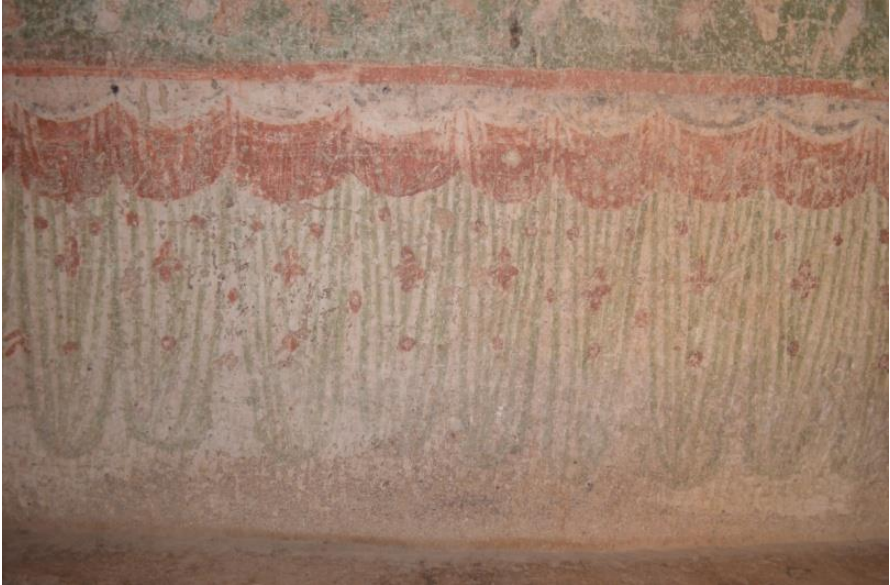
Figure 13: Çavuşin Güvercinlik Church, north wall of naos (M. Kaya, 2017)
