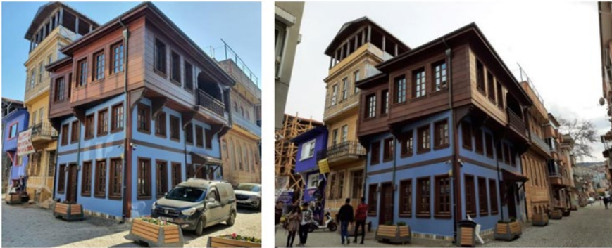
Figure 10. Photos dated 2023 of the structure located on 1448 Island 1 Parcel (The author's own archive)
