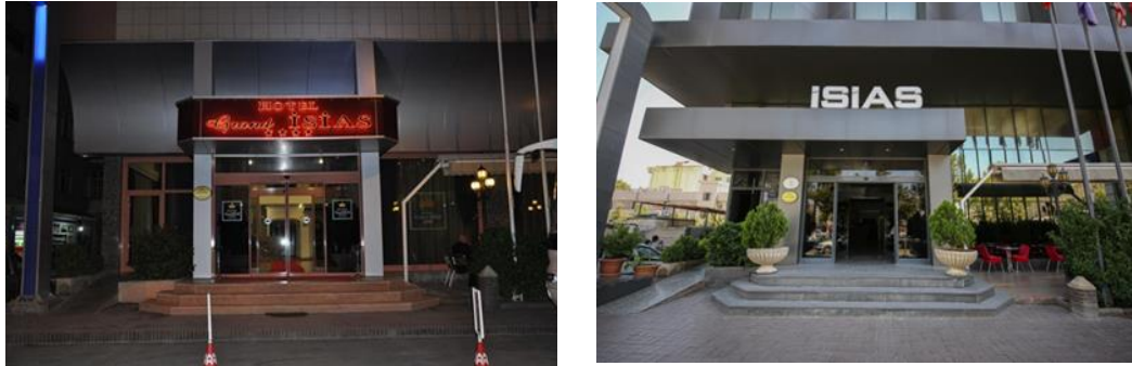
Figure 6. a-b. Hotel entrance after extensive- major renovation (GIO, 2023)
