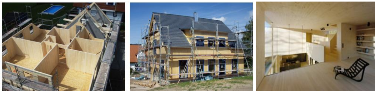
Figure 2. Examples of buildings using CLT panels (Mestek, Werther & Winter, 2010)
