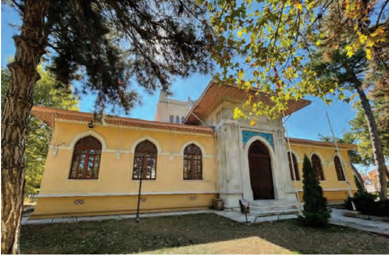
G. 2: Edirne Union and Progress Club Building, Front View (A. Balcı, 2022)
