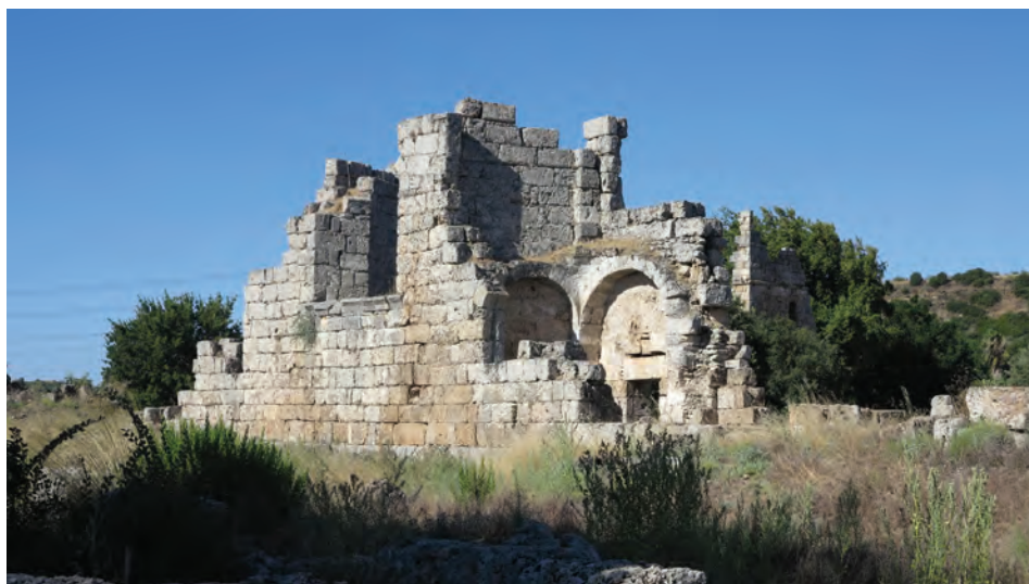
F. 9: The eastern facade of the South Church, view from the northeast (A. Tiryaki, 2022)
