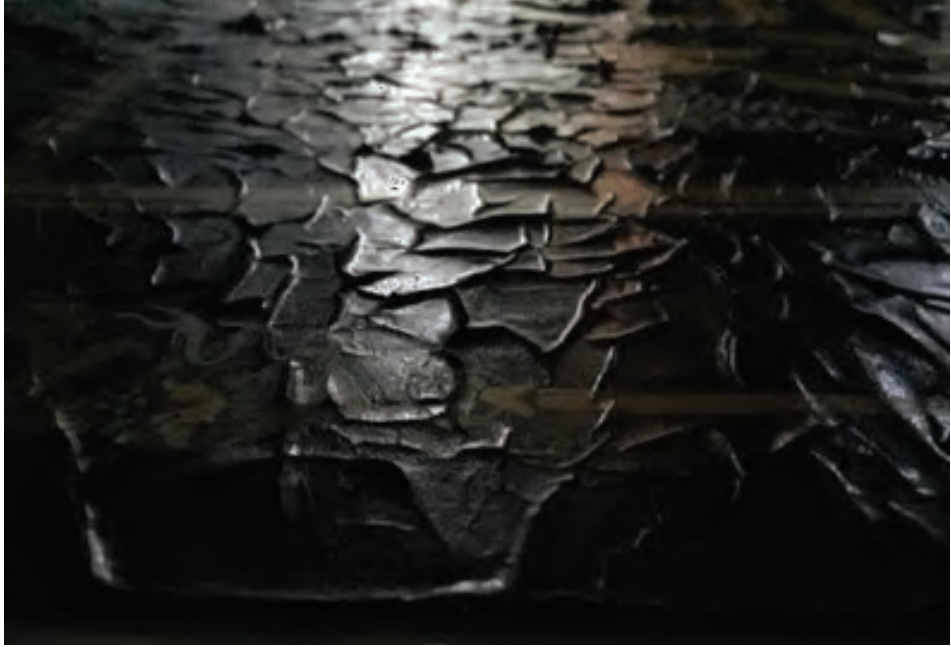
F. 17: Details in visible light (VIS)- Cracks and blisters parts of the paint layer (Gülde Emre, 2019)
