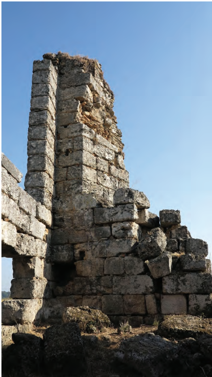
F. 18: The side window of the apse, view from the north (A. Tiryaki, 2022)
