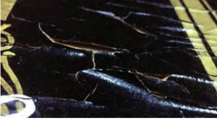
F. 9: Blistering of the paint layer (Güldeir Emre, 2019)
