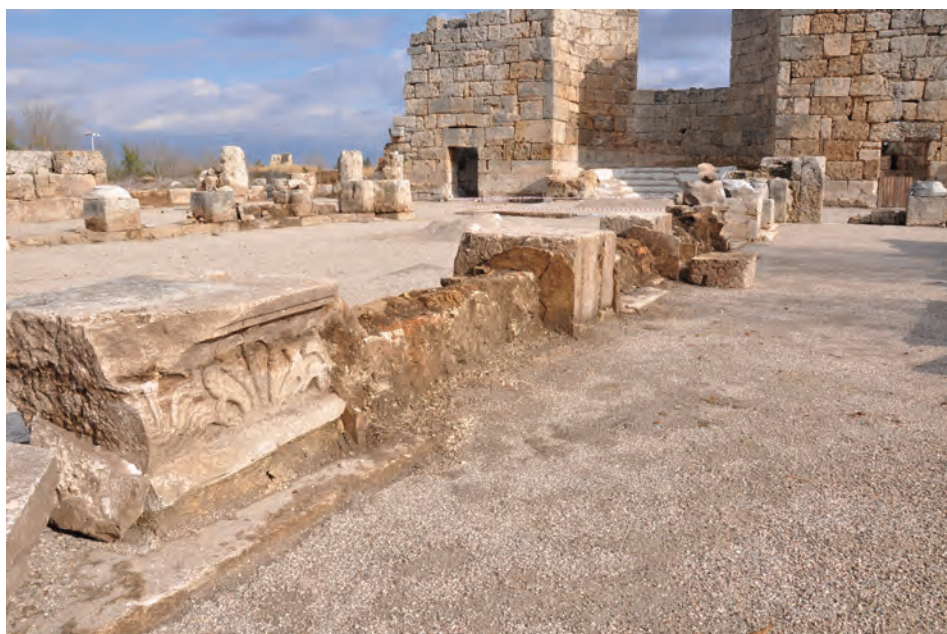
F. 6: The rubble walls on the southern stylobate, view from the southwest (The Antalya Museum Archive, 2016)
