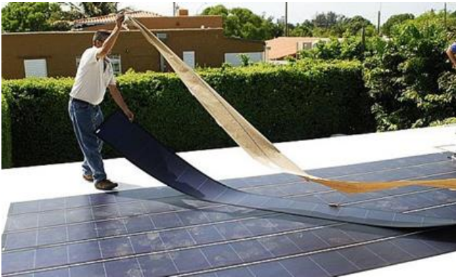
Figure 11. Integration of thin film PV system on roof [20].
