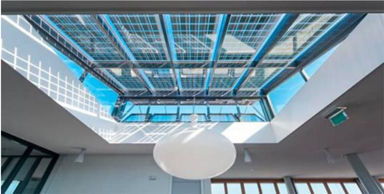
Figure 10. Example of Glass PV system used in buildings [18].
