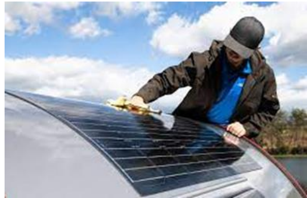
Figure 11. Integration of thin film PV system on roof [20].
