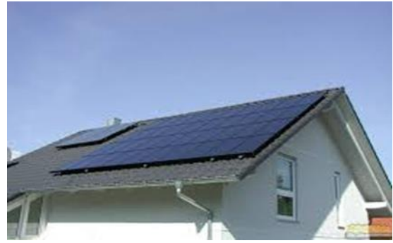
Figure 12. Integration of framed PV systems into the building [21,22].
