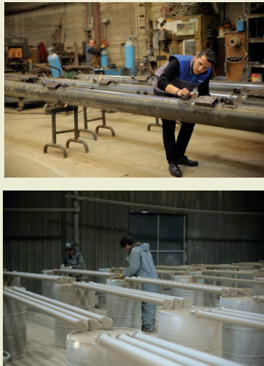
Figure 3. Preparation of S235JR steel construction
