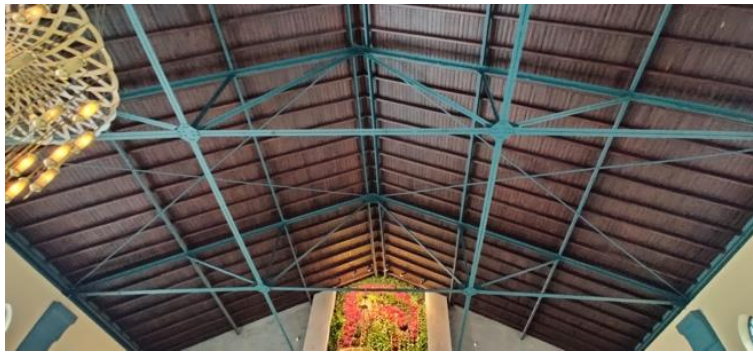
Figure 5. Restored roof structure (Torunbalcı archive, 2019)
