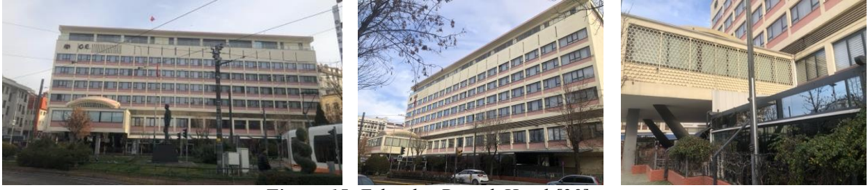
Figure 15. Eskişehir Porsuk Hotel [20]
