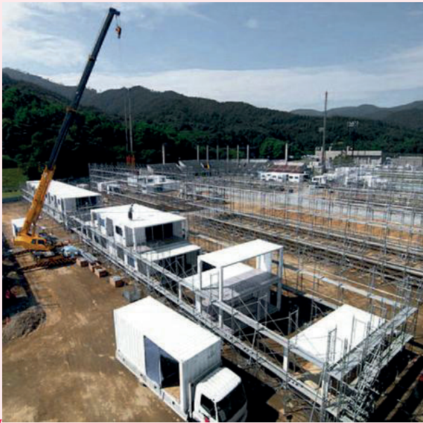
Figure 7. Delivery of Ready Containers to the Region (URL-6, AD: 24 May 2023)
