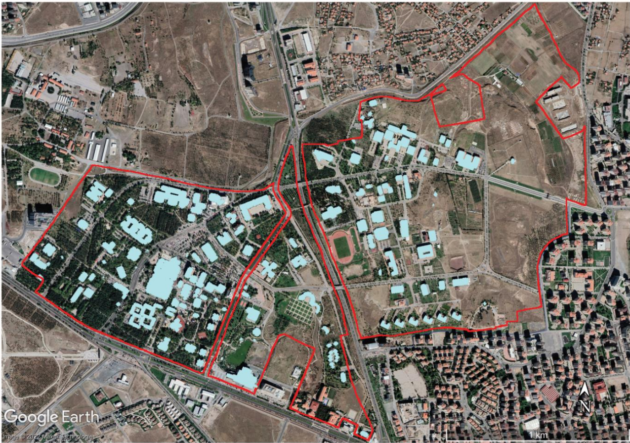
Figure 2. Erciyes University campus boundary and the buildings considered in this study
