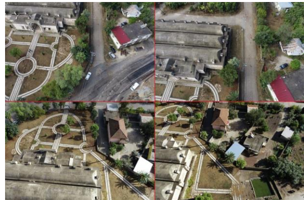
Figure 4. Sample images of Kurtkulağı Caravanserai taken by nadir photogrammetry.
