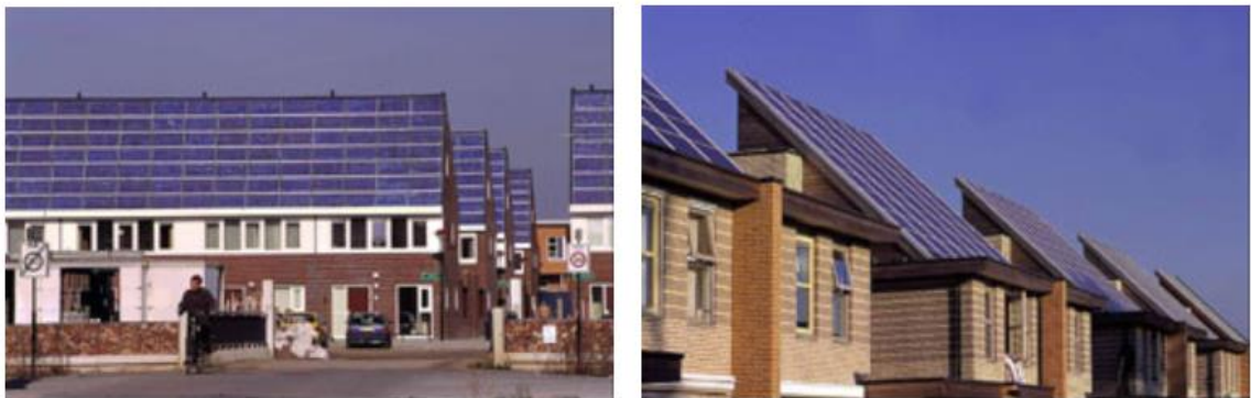
Figure 9. 'Millennium Electric PV/T System (Milenyum Solar, 2023).
