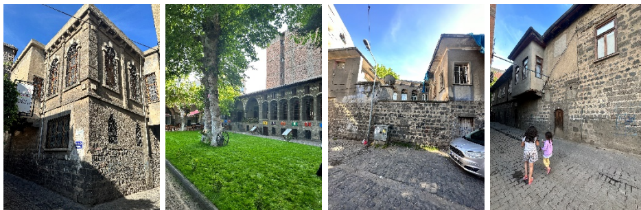
Figure 5: Examples of undamaged structures
