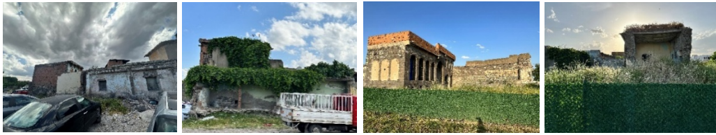
Figure 4: Buildings with minor and moderate damage
