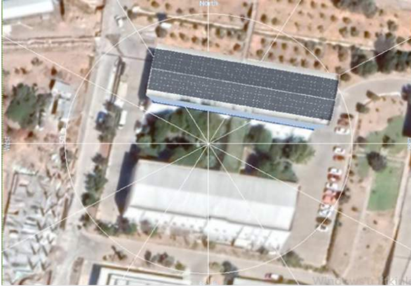
Figure 4. Pitched Roof Panel Installation
