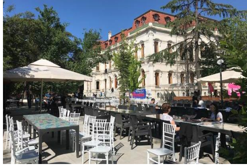
Figure 4. Front garden of Adile Sultan Pavilion, marbled and fenced in the restoration period.
