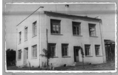
d. Akalan Halkevi Building (Republic of Türkiye Presidential State Archive (CDA) 1691 - 876 - 1 / 00.00.1943-16.05.1945 / no: 37, 1945i)
