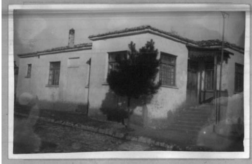
a. Kızılca Halkevi Building (Republic of Türkiye Presidential State Archive (CDA) 1691 - 876 - 1 / 00.00.1943-16.05.1945 / no: 33, 1945e)
