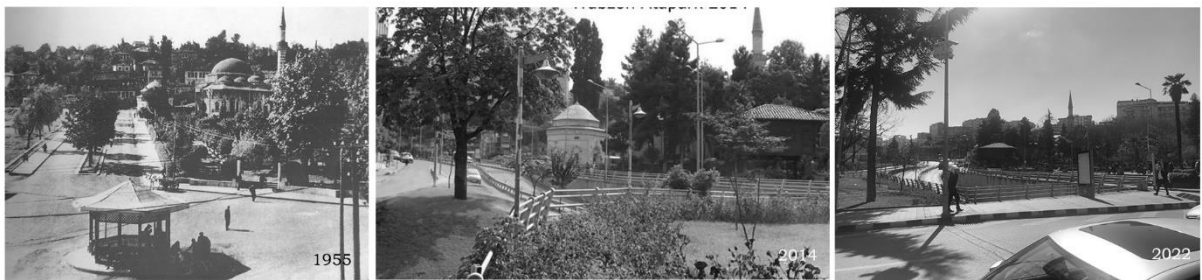
Figure 12. The weakening of the building-city relationship of Gülbahar Hatun Mosque (Bölükbaşı, 2006; Bayram, 2022)
