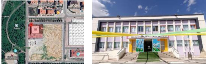
Figure 5. Location and entrance facade of Selçuklu Sabir Kindergarten (Google Map,2023; Sungur, 2023)
