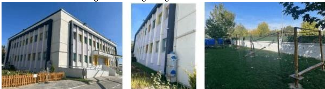
Figure 7d. Stairs and ramp providing access to the building, rainwater collection tank, wooden play equipment
