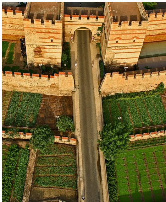
Figure 13. The photo of triple defense system of the Theodosian Walls (Istanbul Site Management Unit, 2020)
