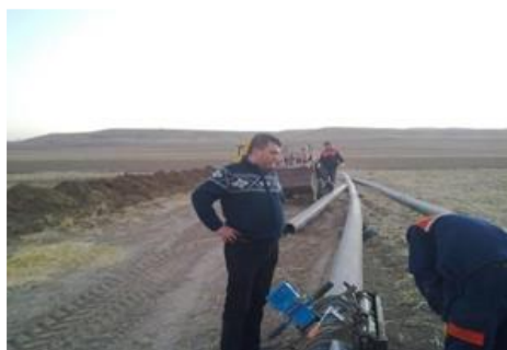
Figure 6. PE 100 pipes and jointing works by butt welding method
