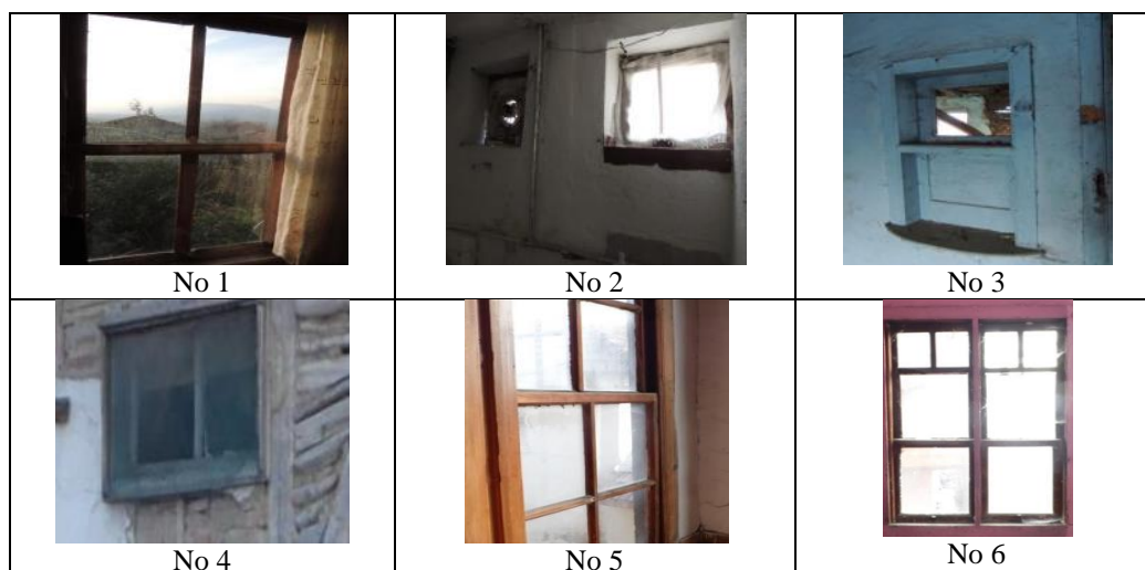
Figure 14. Windows of Houses No. 1, 2, 3, 4, 5, and 6
