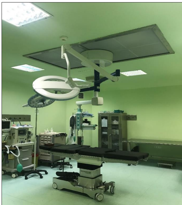
Figure 1. Laminar airflow (LAS-OR) system.
