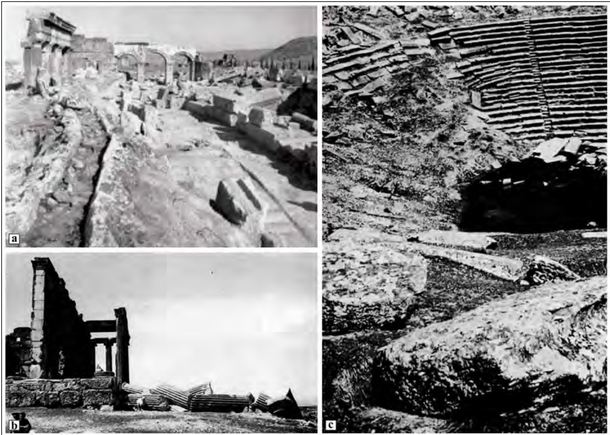
Figure 6- a) Photo presented in D'Andria et al. (2008) showing the deformations that occurred during the 7 th century earthquake on the Plateia (city square) extending to the Frontino Gate, which was taken during the 1963 excavations in Hierapolis. Some photos in Rudolf Naumann's work documenting damage after the March 28, 1970 Gediz Earthquake in the ancient city of Aizanoi; b) systematic aligned fallen columns of the Temple of Zeus, c) deformations in the cavea of Theater and lateral displacements in large buried marble blocks.
